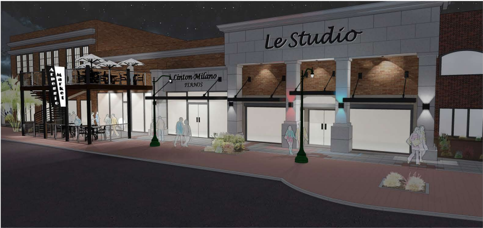
VIEWING SOUTHEAST AT NIGHT
